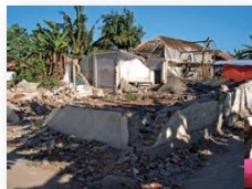
Collapsed houses in Klaten ©ICA/JPF
