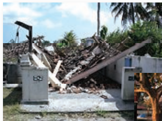
A collapsed house in Java ©JPF
