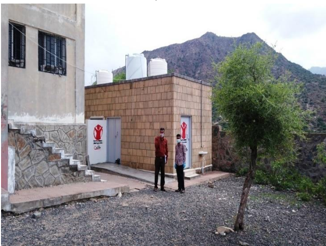
Latrines at 30 November School, Al-Mafalis area, Hayfan, captured by MEAL Center field staff, September 10, 2022
