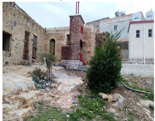
Incinerator and latrines at Al-Faqeed Mansour Ahmed Said School, As Silw, captured by MEAL Center field staff, September 14, 2022
