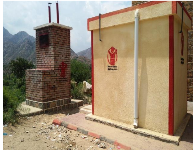
Incinerator at Omar Ibn Al-Khatab School, Al-Mafalis area, Hayfan, captured by MEAL Center field staff, September 11, 2022
