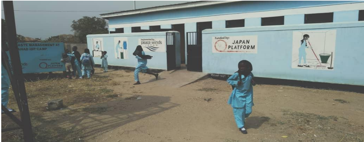
Figure 9: Permanent latrine in Mahad IDP camp constructed by the project
