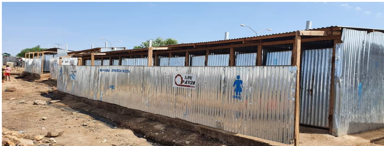
Figure 10: semi-permanent toilets reconstructed by the project
