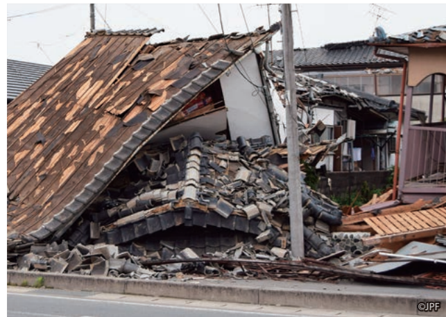
A destroyed house in Mashiki
