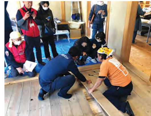
Floorboard removal at a house preservation workshop ©PBV
