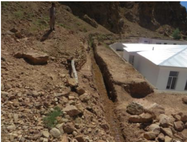
Figure 20: There is risk of flooding and damage to Abdara school building.
