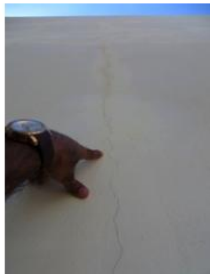
Figure 25 and 26: Cracks on the walls of newly constructed building. The cracks have been painted with the same color of the walls the day before our visit.
