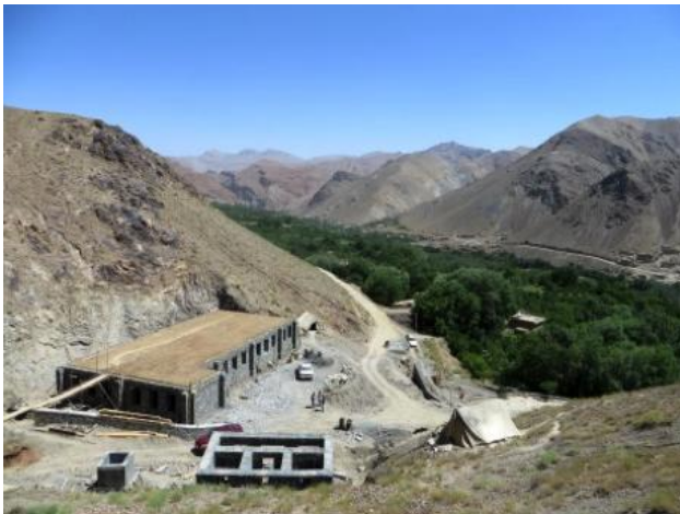
Figure 12: The new Gunbad village school building under construction (JPF funding).
