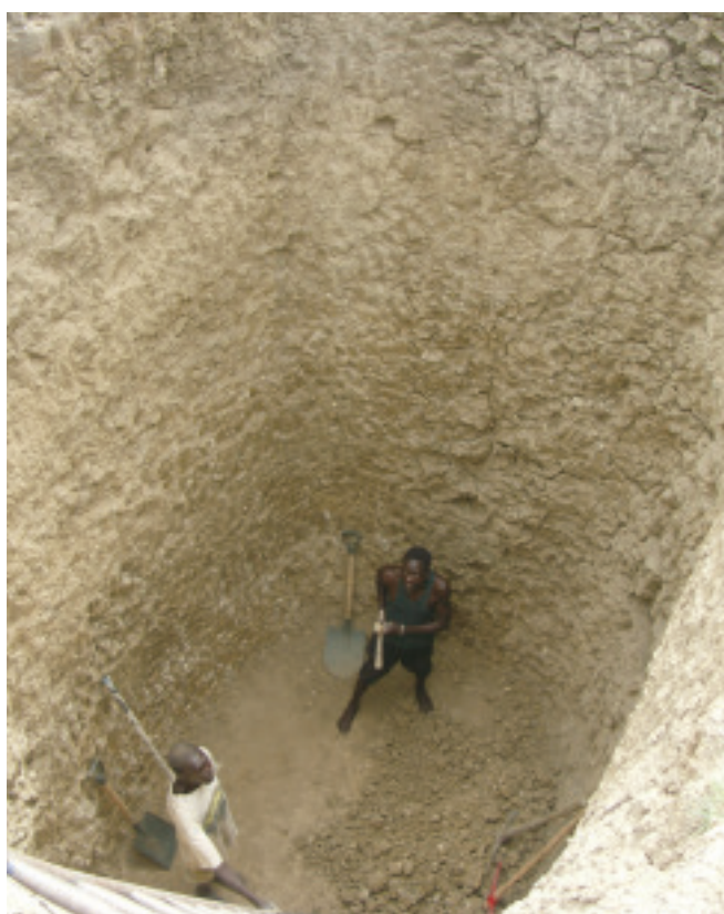
A latrine pit dug by local residents
