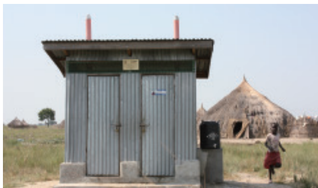
Public latrines constructed at a primary school
